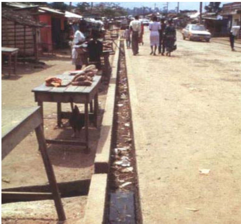
An open sewer along a roadside market in Ghana
